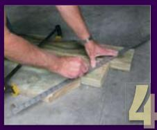
**Lay three different**-sized boards side by side with spacer in between. Extend the 30° line from the first board to the second two.
