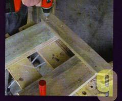
With an 8mm drill bit, drill four clearance holes right through braces and legs. Drill on diagonals, as shown.
