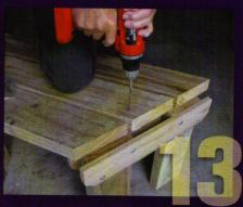
Carefully stand upright (they're not properly secured yet). Mark a screw line at centre of braces. Screw boards in place.
