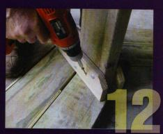
**Drive screws diagonally** through legs and into the underside of seat. Repeat steps 11 & 12 to make up another section.
