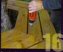
Once level, adjust seat sections so they're one seat board length apart. Drop in remaining planks and secure with screws.
